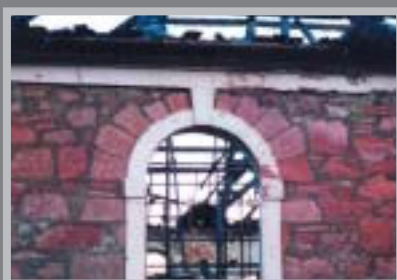
The building after an extensive fire gutted the former church in 2000. The charred roof timbers remain in place; allowing the roof to be reconstructed to the original profile.
