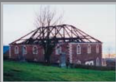
The building after an extensive fire gutted the former church in 2000. The charred roof timbers remain in place; allowing the roof to be reconstructed to the original profile.
